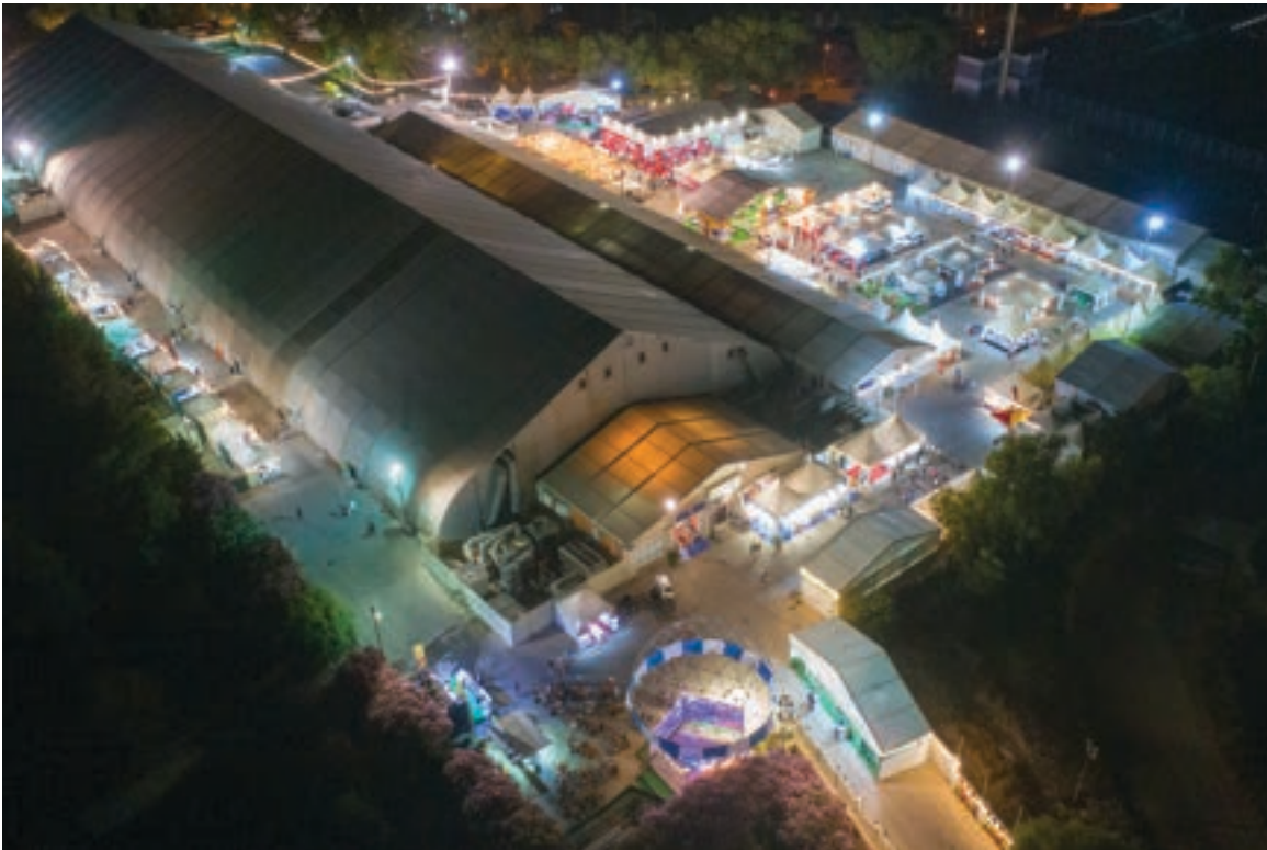
TENSION FABRIC STRUCTURE (TFS) AND GROUNDS
